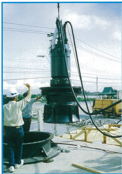
VERTICAL SUSPENDED COLUMN WITH VERTICAL DISCHARGE
