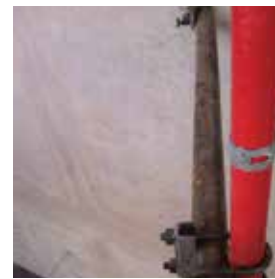
PT. UNILEVER Sismic Bracing Tolco Medan
