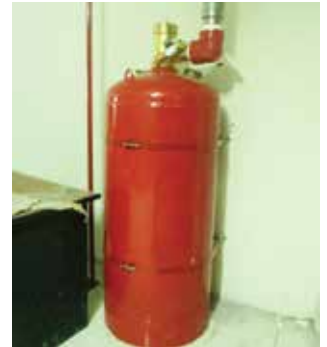
BANDARA NGURAH RAI Gas Fire Suppression Sapphire System Bali
