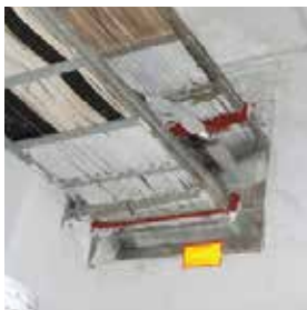
PINDO DELI Fire Passive - Fire Stopper Karawang
