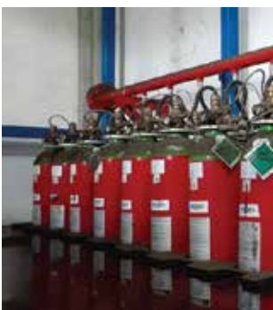
LRT PANBEK Gas Fire Suppression Inergen Flow Jakarta
